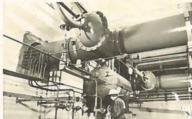
The Nordarmatur Group manufactures and markets amongst others valves for power plant. NAF wedge gate valves has been installed in the Oskarshamn nuclear power plant.
